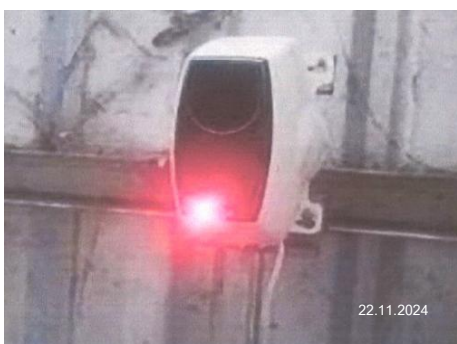
Smoke Beam Detector
